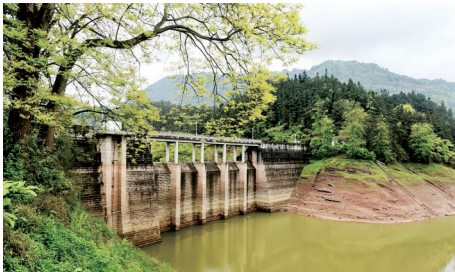
清溪沟水库大坝
